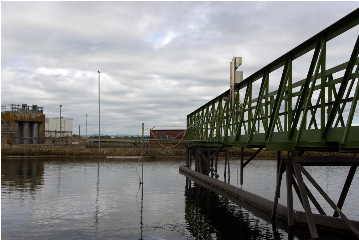
Figure 4 Avocet-9000 Outstation Installation
